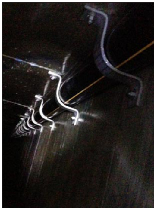
HORIZONTAL PIPE SUPPORTS
