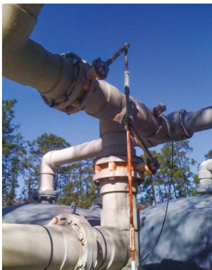
IMAGES 1 & 2 (before, left; after, right): Over 20 years ago, the Typhoon Lagoon Waterpark at Disney World in Orlando, Florida, experienced corrosion issues on the metallic valves in their water filtration system. Thermoplastic Type-57LIS valves were provided as a direct metal valve replacement. The valves are still operational and problem-free as of today. (Images courtesy of Asahi/America, Inc.)
