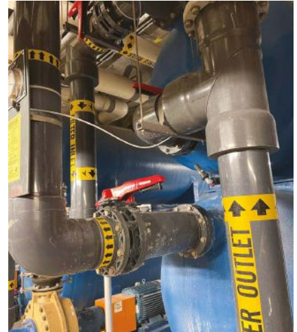
IMAGES 3 & 4 (before, left; after, right): In 2013, Mandalay Bay in Las Vegas replaced a majority of the corroded stainless steel valves in their shark reef exhibit with these 6-inch and 8-inch Type-57LIS butterfly valves. The valves are still operating without issues in their saltwater sand filtration system.
