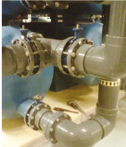
IMAGES 3 & 4 (before, left; after, right): In 2013, Mandalay Bay in Las Vegas replaced a majority of the corroded stainless steel valves in their shark reef exhibit with these 6-inch and 8-inch Type-57LIS butterfly valves. The valves are still operating without issues in their saltwater sand filtration system.
