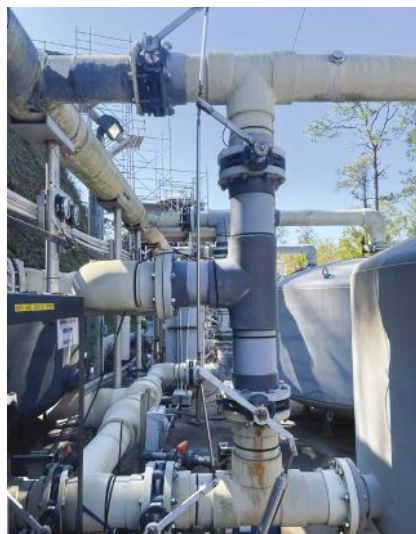
IMAGES 1 & 2 (before, left; after, right): Over 20 years ago, the Typhoon Lagoon Waterpark at Disney World in Orlando, Florida, experienced corrosion issues on the metallic valves in their water filtration system. Thermoplastic Type-57LIS valves were provided as a direct metal valve replacement. The valves are still operational and problem-free as of today. (Images courtesy of Asahi/America, Inc.)
